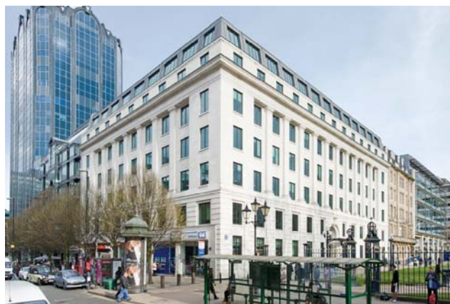
Figure 2: 5 St Philip's Place, Birmingham
